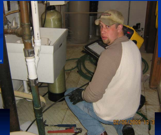
Inspector with Push Camera
