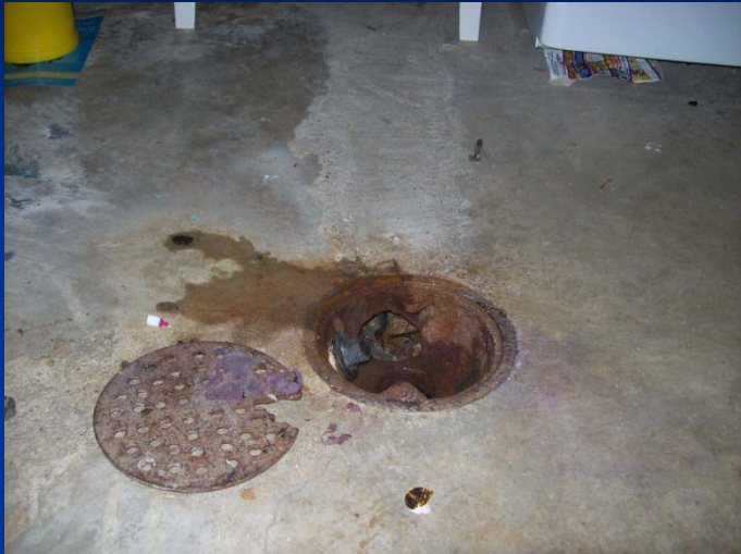
Foundation Drain – Floor Drain
