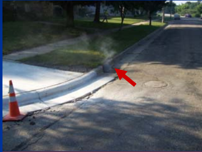
Inlet Inflow - 7 th and 10 th Ave SE
