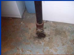
Inaccessible – Clean Out In Concrete
