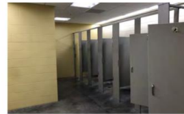
Womens Toilet Room
