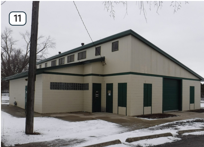
West shelter building*
