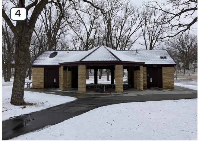
East shelter building*
