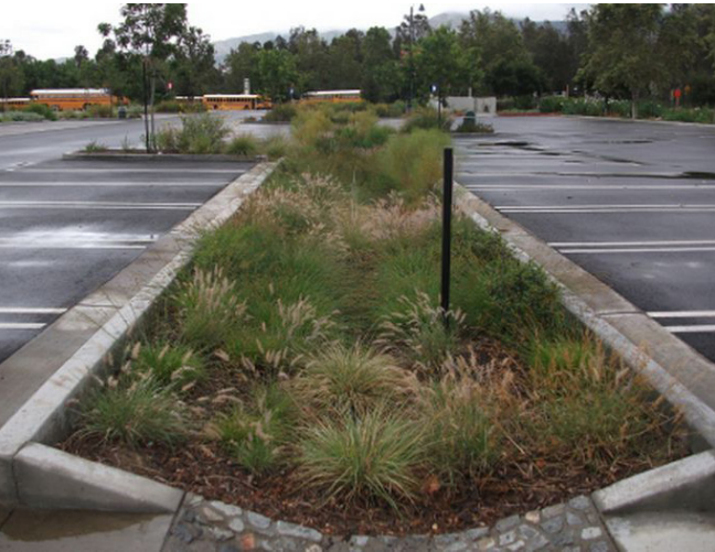
Bioswale in Parking Lot
