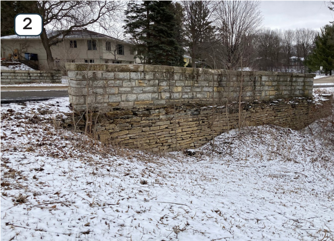
2 East stone wall*
