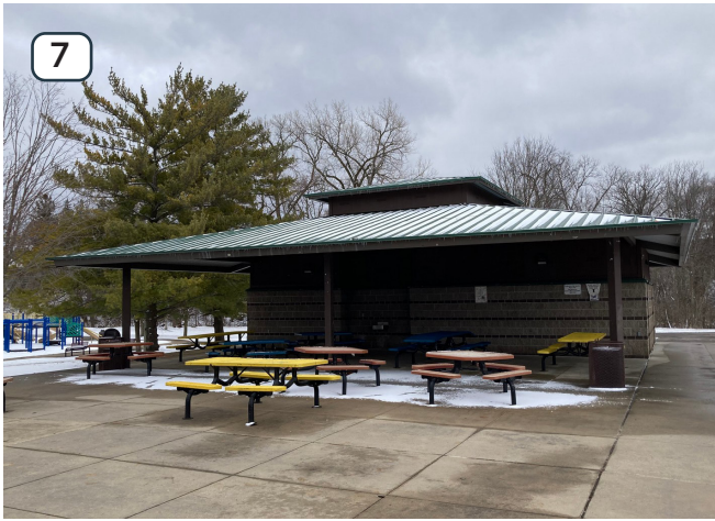
South shelter building
