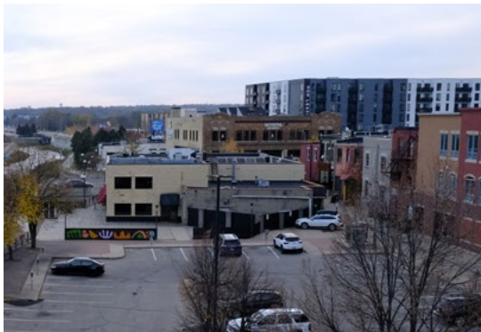
Left: View of North facade of Red Owl + Time Theater building from parking garage, existing conditions in December 2021.
