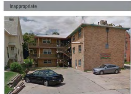
No transitional element at building entrance
