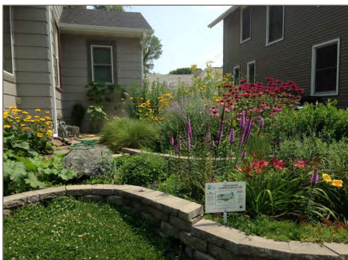
Rain gardens treat stormwater at its source. Source: Rochester Public Works
