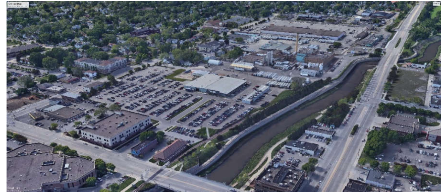
Figure 9: View of DWSE Project Area Looking Southeast
