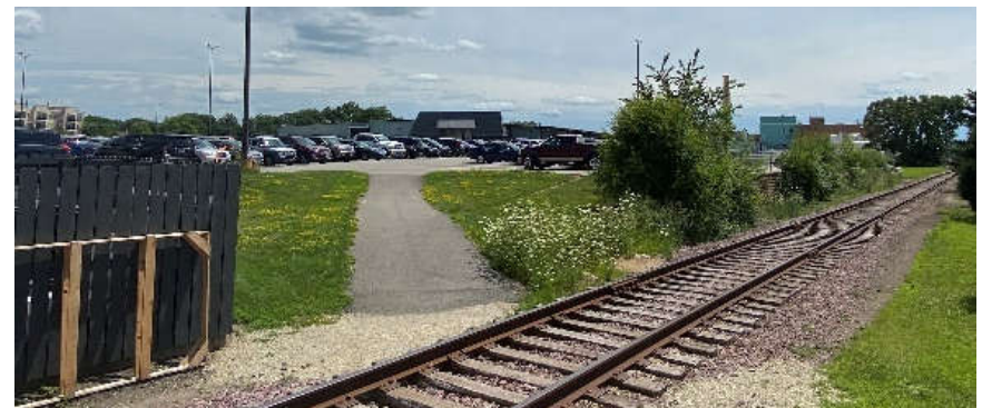
Figure 14: View of the CP/DME Rail Spur and the Fullerton Commuter Parking Lot Looking Southeast from 4 th Street St
