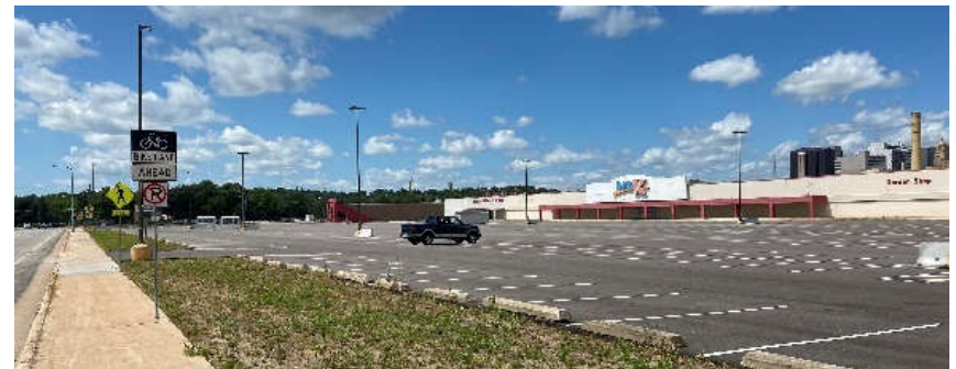
Figure 13: View of Former Kmart Looking West along 9 th Street SE
