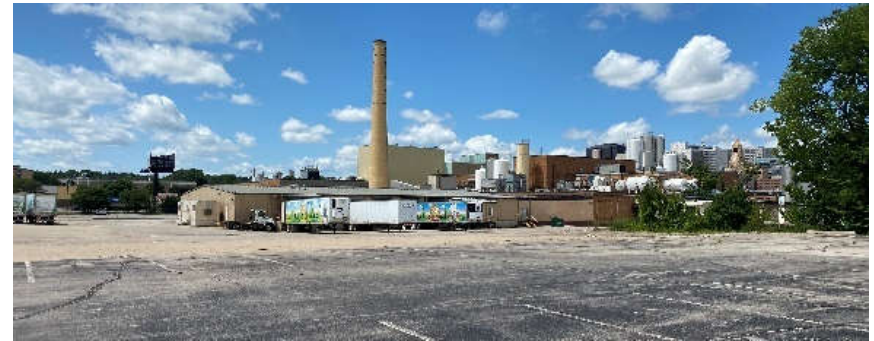
Figure 12: View of the Former AMPI Facility Looking West from 3 rd Avenue SE
