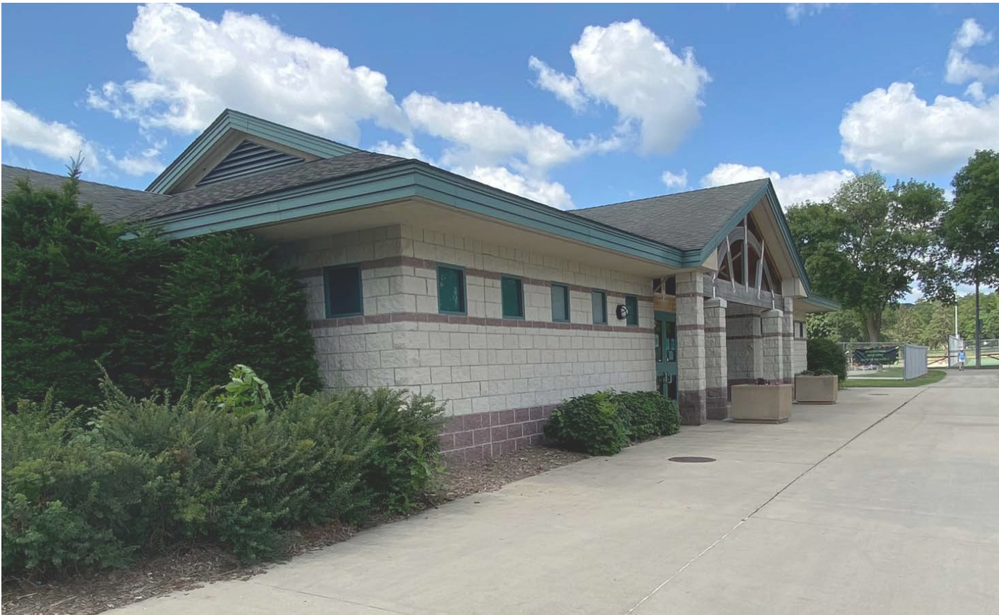
Existing bathhouse and aquatics facility entry
