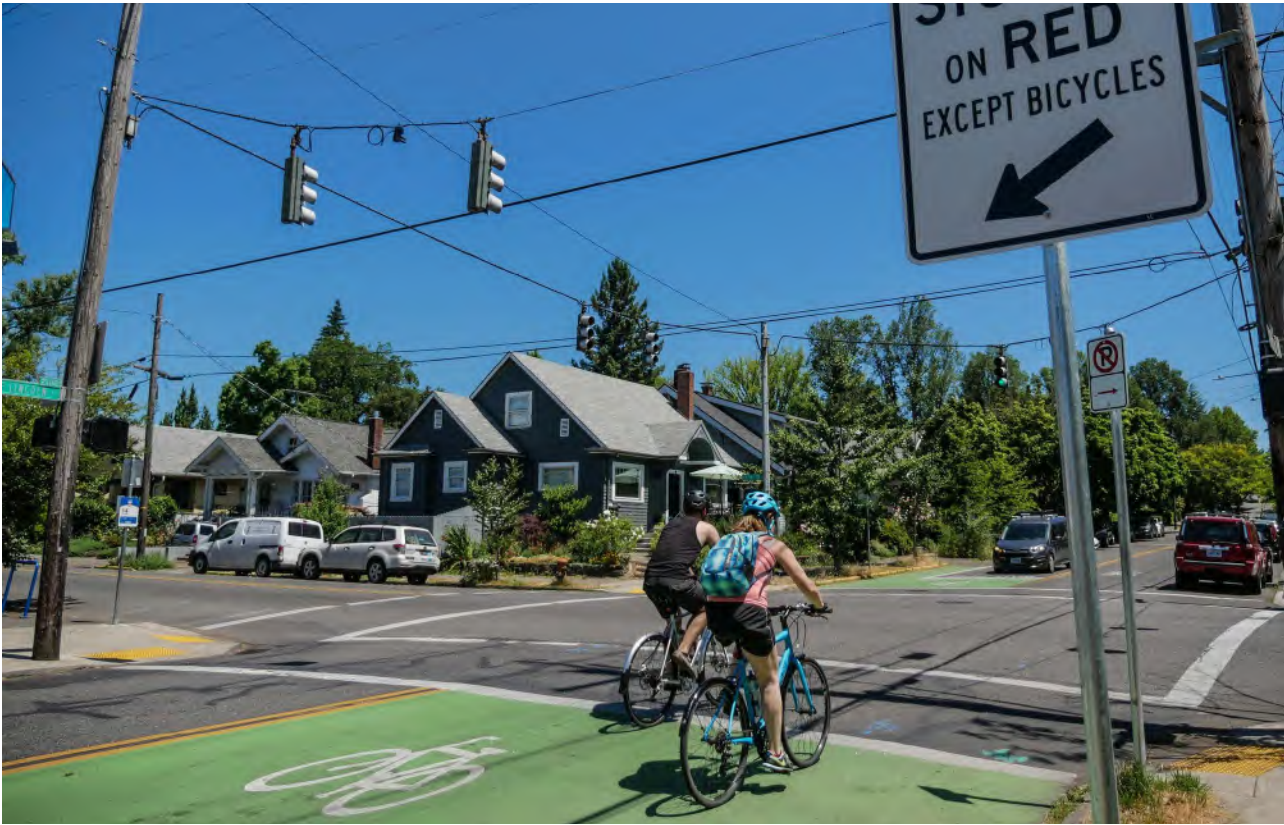
A bike box allows for bicyclists to wait in front of queuing traffic, providing high visibility and a head start over motor vehicle traffic.
