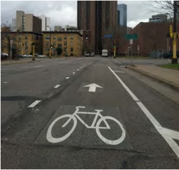
A recessed thermoplastic bike lane marking in Minneapolis, MN.
