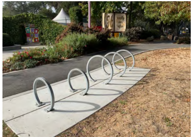
Racks with square tubing, good spacing, and a concrete base likewise offer two points of contact.
