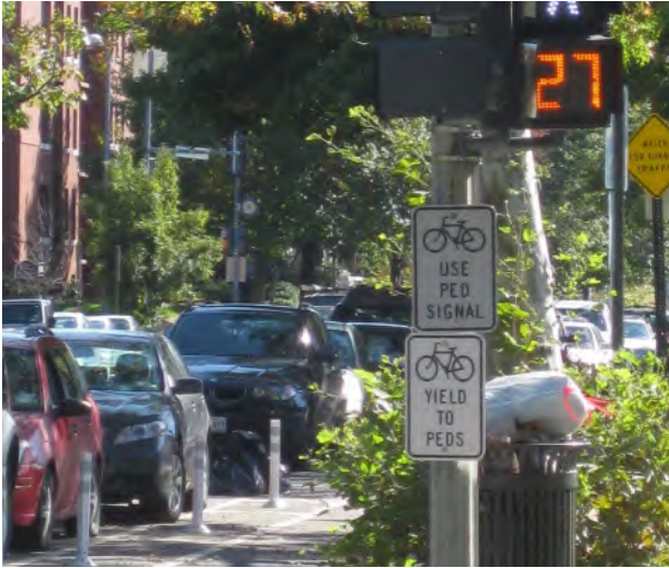
A bicycle signal head at a signalized crossing creates a protected phase for cyclists to safely navigate an intersection.
