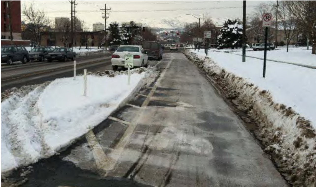
A parking protected bike lane in Salt Lake City, UT after a snow plow operation. Photo Credit: Travis Jensen
