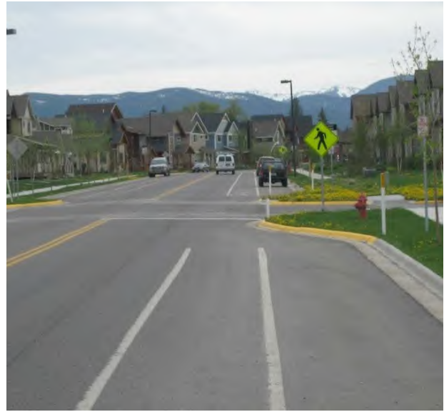
Vertical delineators help inform snow plow drivers of obstacles such as cycletracks, raised medians and bulb-outs in Bozeman, MT.
