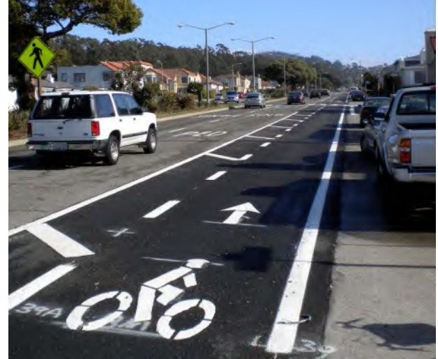
The use of additional pavement markings delineates space between vehicles and bicyclists.
