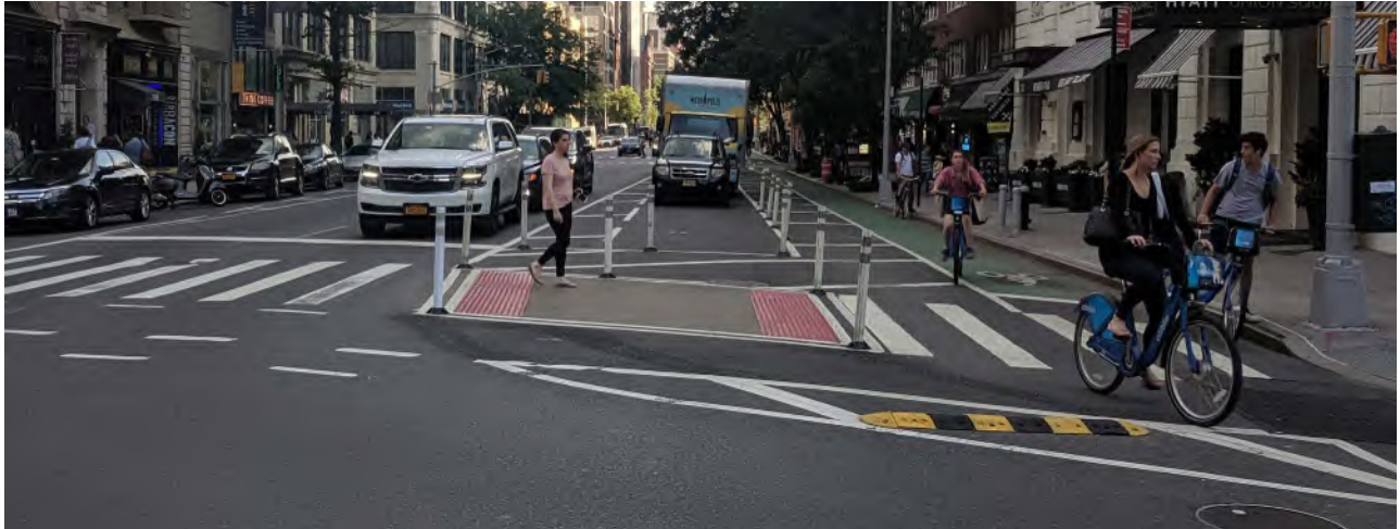
Parked cars serve as a barrier between bicyclists and the vehicle lane. Barriers could also include flexible posts, bollards, planters, or other design elements. Source: Alta
