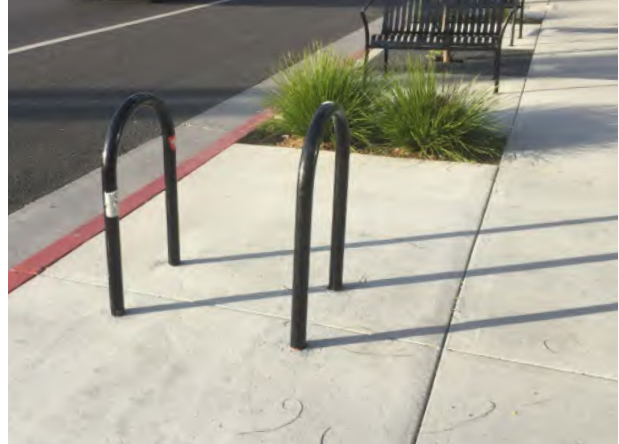
Inverted-U racks provide two points of contact.
