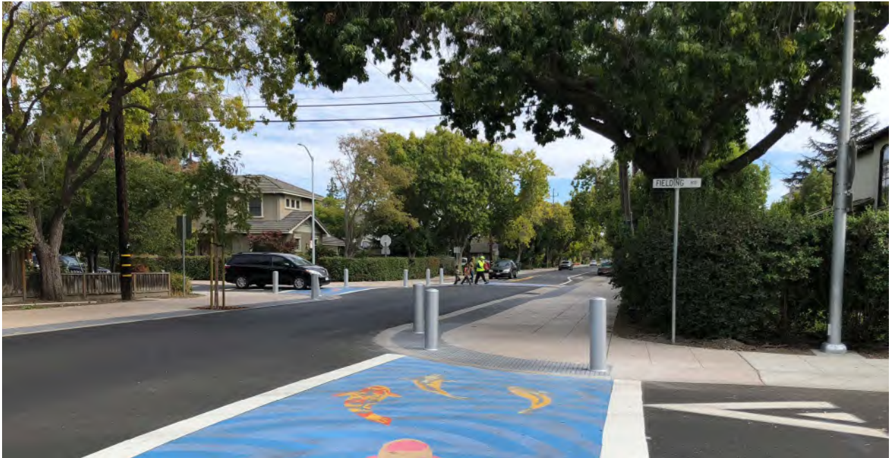
Unique crosswalk markings can be used to draw attention to the raised intersection, as demonstrated above on an offset residential intersection.
