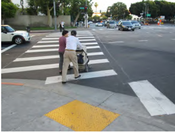
Not recommended: Diagonal curb ramp configuration.
